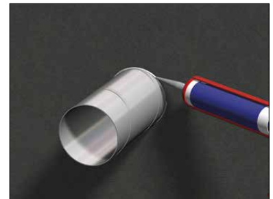
D6. Jointing around lead-throughs
